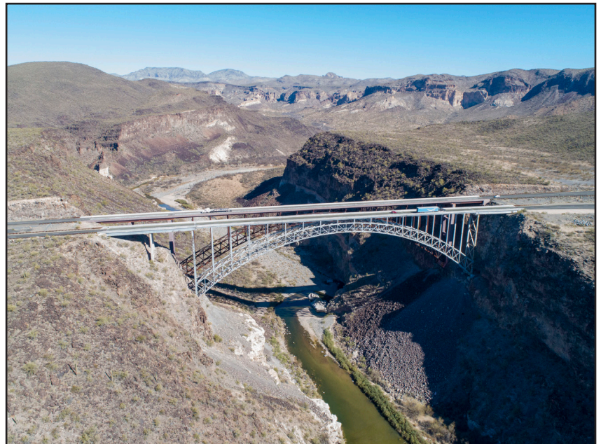
Figure 26. Aerial drone view looking north at US Hwy 93 bridge over Burro Creek towards the Kaiser Springs volcanic field. Elephant Mountain is visible on the horizon-left.
