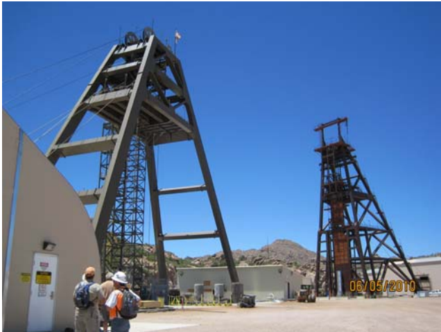
The new No. 10 headframe (left) and the No. 9 headframe. The No. 10 shaft is being advanced at a rate of about 10 feet per day.
