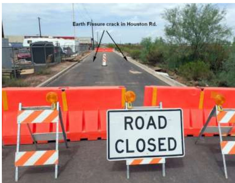
Figures 1a-b. W. Houston Road closed due to damage from earth fissure. Earth fissure nicely exposed adja- cent to W. Houston Rd. Photos by Joe Cook.
