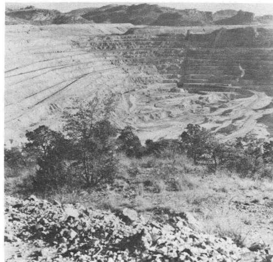
Figure 14 – Chino copper mine of Kennecott Copper Corporation – largest mine in New Mexico. Note skip–haulage system on far wall. Hills in background are of Tertiary volcanic rocks (mainly Kneeling Nun Quartz Latite ash-flow tuff) which unconformably overlie the mineralized Laramide porphyry body. Much of the oxidation and secondary enrichment is pre-volcanic, and preserved from erosion by the volcanic rocks that once blanketed the ore body. –Photograph by W.E. Elston
