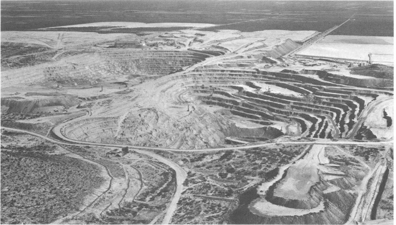
Figure 1 — View from the west looking eastward toward Santa Cruz Valley. Pima Mine nearest and on the right and ASARCO's Mission Mine on the left. Note displacement of benches within slump pattern in the Pima pit. —Photograph by Tad Nichols
