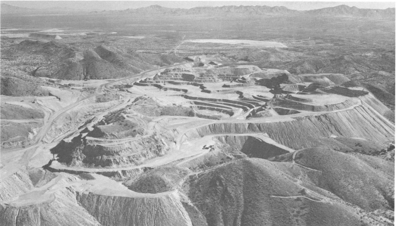
Figure 2 – Esperanza Mine viewed from the west in January 1968 looking across the Santa Cruz Valley toward the north end of the Santa Rita Mountains on the skyline. Tailings pond in the middle distance and Twin Buttes development near the top-left portion of the picture. Sierrita development to take place in ground of bottom-right portion of photograph. –Photographs by Tad Nichols
