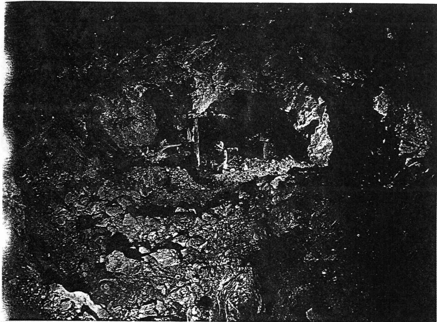
Figure 24. A portion of a stope in the Copper Queen mine, excavated in the 1880's.
