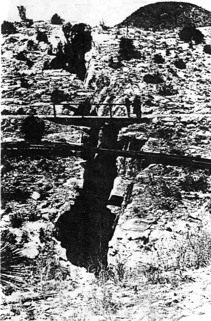
Figure 10. Surface fissures formed by subsidence due to the oxidation and later mining of copper deposits below, in the Copper Queen mine.
