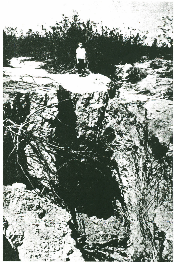
Figure 5.—Magnitude of fissure opening near Chandler Heights, viewed from site marked by arrow A in figure 4A. Photographed on September 16, 1961, by D. E. Peterson.
